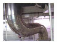
All lagging should be free from oil, grease or other flammable contaminants and maintained without exposed hot surfaces.
